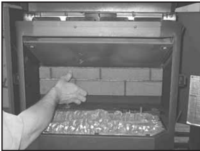
Figure 8.5 Install rear panel, gently wedging it between support shelf and baffle base. Install the brick brackets that are enclosed with the brick set.
